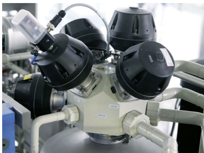
GEMÜ M-Block with electro-pneumatic positioner GEMÜ 1434 µPos
